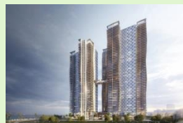
WYNDHAM SOLEIL Son Tra District Under-construction
